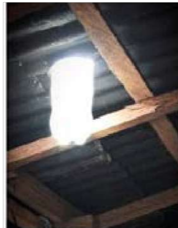
Using plastic bottles on the roofs which capture sunlight will be used in order to provide natural daylight. Photo credit: instructables.com
