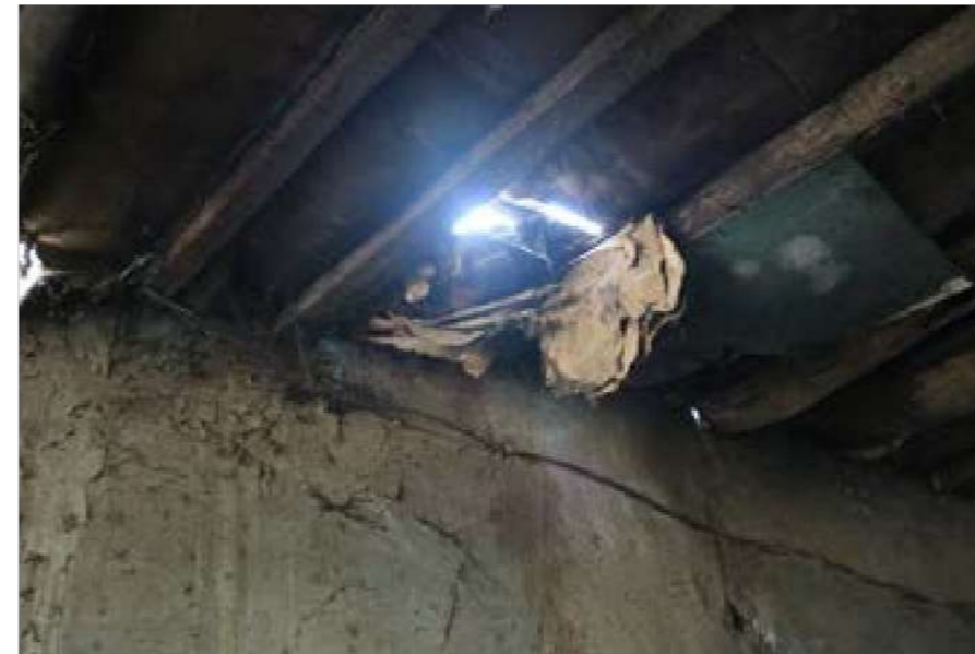
A hole in the ceiling made of cardboard in the house being redesigned. Photo credit: Hand Over team
